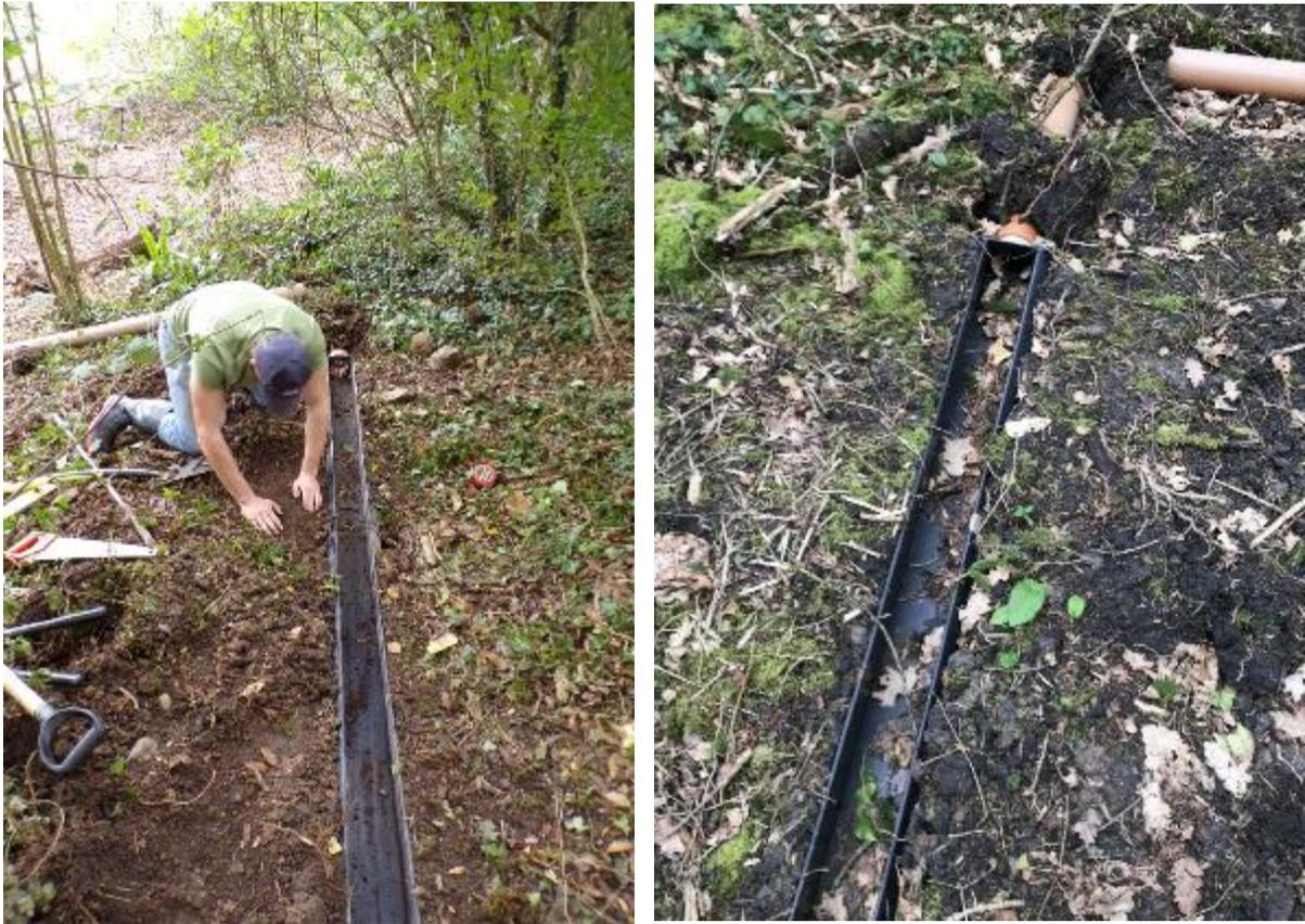
**Figure 20** Guttering embedded at the soil surface to capture downslope runoff
