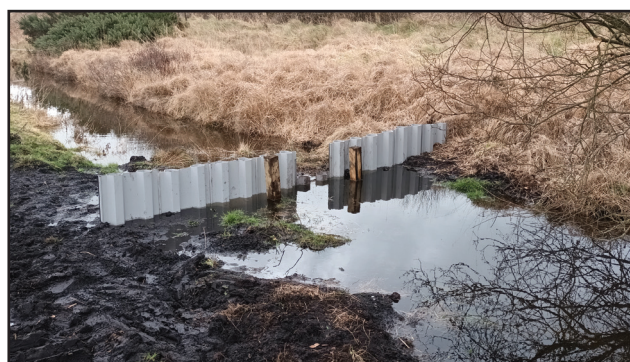
Drain one week after installation of dams
