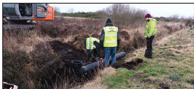
Plastic dam being installed on Case Study Farm A on 7th Feb 2023
